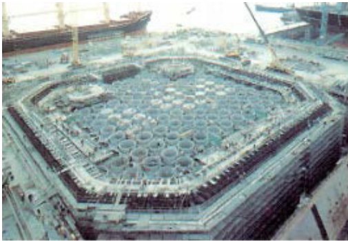
FIG. 1 HONEYCOMB FLOATING STRUCTURE USING UHPC
