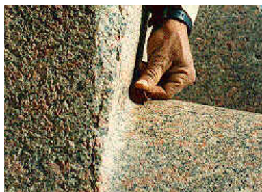
Fig.3 Filleting corners of granite mating surfaces [11].
