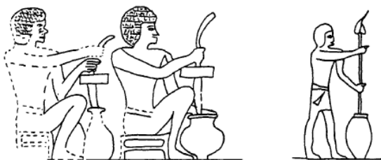
(a) Short-shaft boring drill (18 th dynasty)
