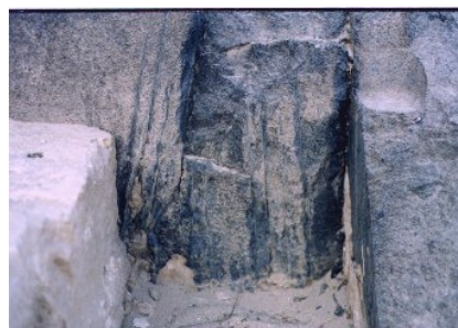
Fig.6 Straight cuts of basalt using stone saw [14].
