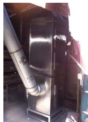
Figure: 7 Packed Bed Scrubber
